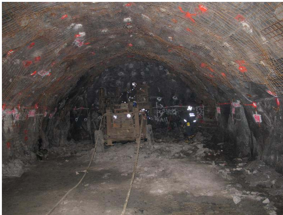
Figure 14 Excavation in the Ladder Labs. Top: Ladder Lab Access Drift. Bottom: The Large drift of the Ladder Labs. This is the top bench and is 4m above the finished floor level.
