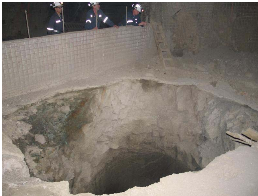
Figure 15 Excavation of the ventilation raises. Top: The raise bore which drills the 3m diameter ventilation shaft. Bottom: The top of the ventilation shaft on the 6600 L of the mine.
